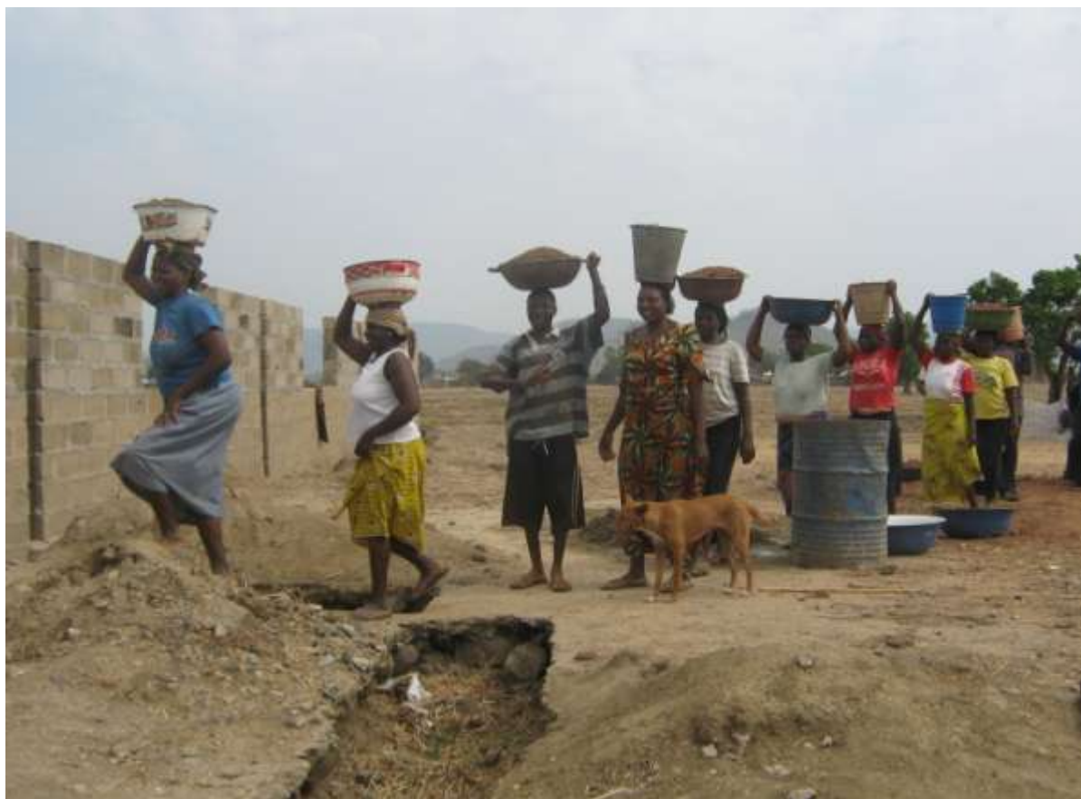
Irchip community at work on their multipurpose town hall project
